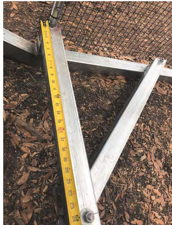
Figure 3: Measure 24" from center of the corner along the end brace and the skid.
