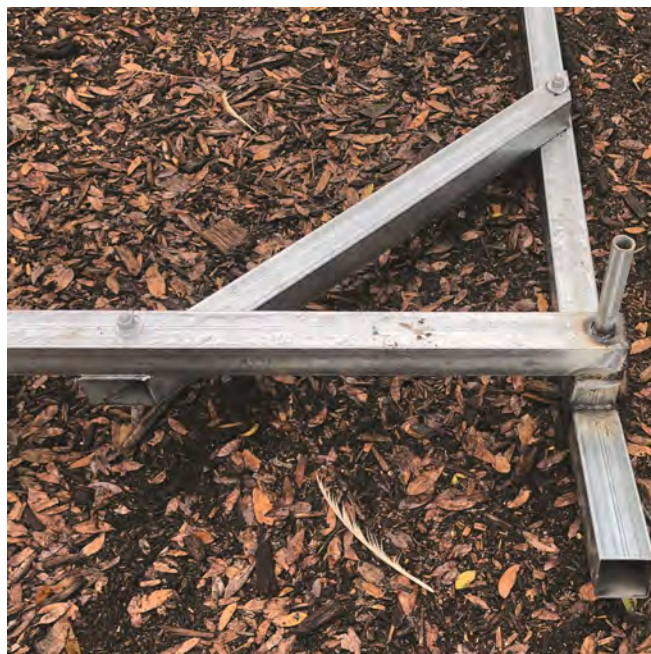
Figure 2: A finished corner showing the 2-1/2" tube stock skid with the corner brace. The pipe nipple is attached to the corner to receive the hoop.
