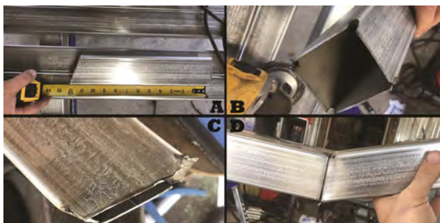
Figure 6: If you're unable to bend the 2-1/2" square stock to form an upturned runner, you can design and weld the end piece of the skid to bend upward at a 22.5 degree angle.
